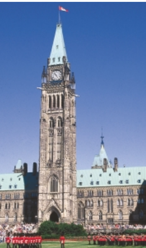
Figure 4.13 When copper corrodes, it turns green. Silver corrosion is black. Which metal was used on the roof of the parliament buildings?
