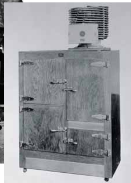
Figure 15.7 An early refrigerator. The compressor is on the top.
