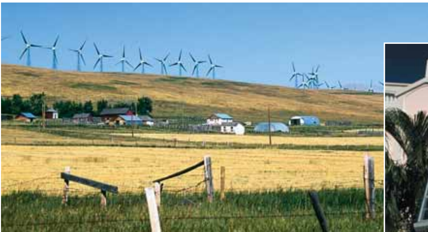
Figure 7.25 For years, windmills have powered water pumps and ground flour. Recently, new styles of windmills have been put together on wind farms. These batteries of windmills produce electricity. The Cowley Ridge Wind Plant, for example, produces more than 55 million kW•h of electricity per year. That is enough to power 6800 efficient homes.
