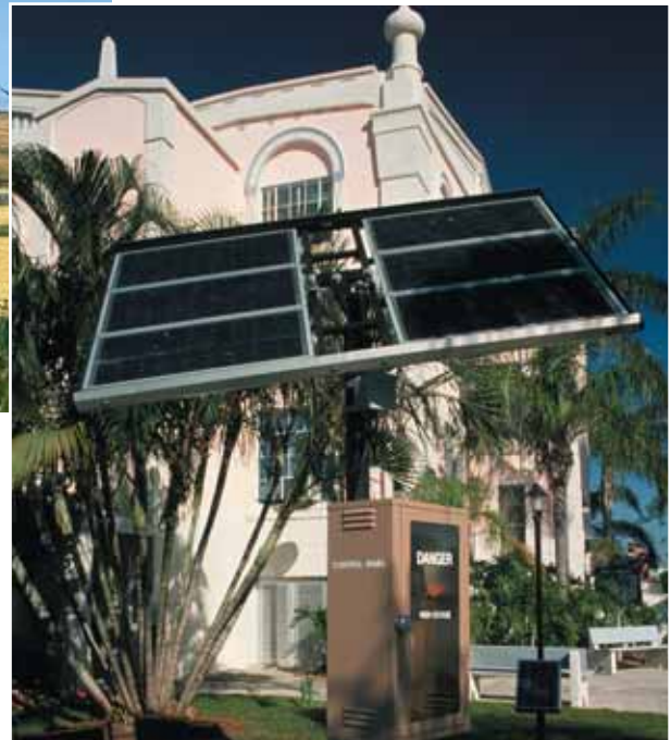
Figure 7.26 Solar panels collect energy from the Sun and convert it to electrical or heat energy. Many Canadians use such panels to run electric fences, heat water, and power calculators and lights. Electricity can either be used right away or stored in batteries for later use.
