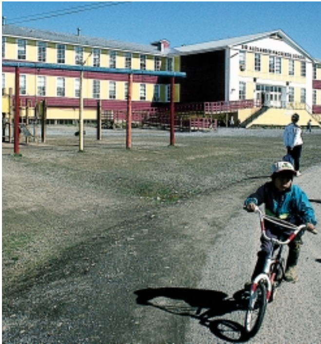
Public buildings have many places where heat loss can occur.
